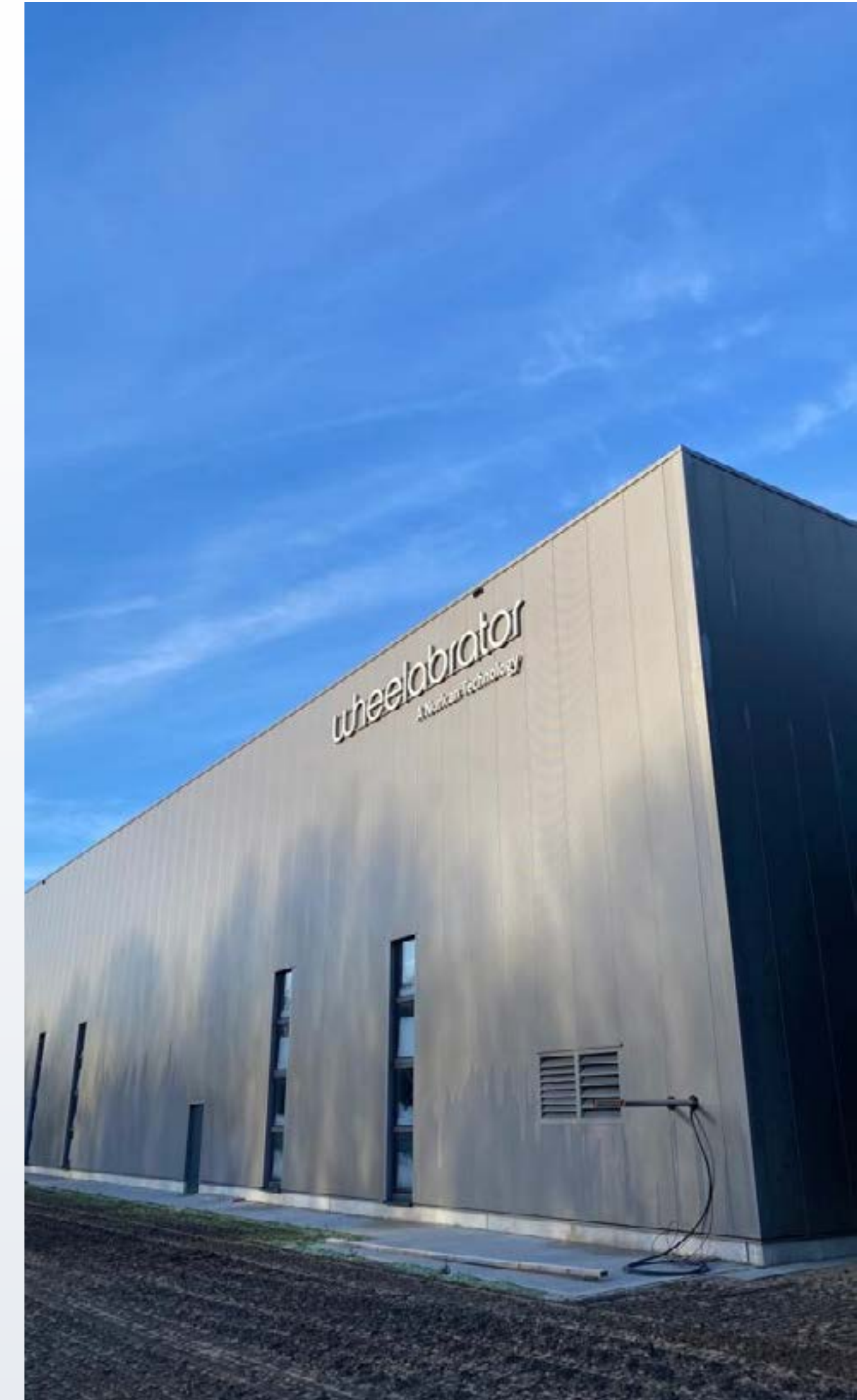
Above: Metelen, Germany
